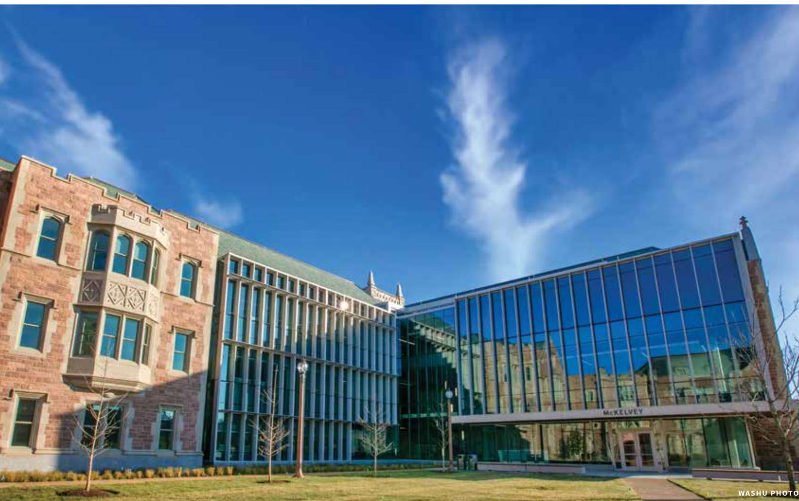
A view of McKelvey Hall from the west. An aluminum and glass curtain wall is used to flood the building with natural light.
